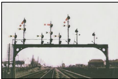
left: The signal gantry at South Ruislip on the approach to Northolt Jn East.
